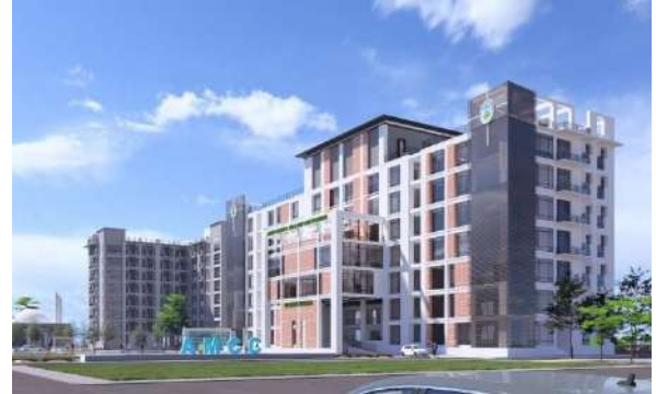
Permanent Campus (Under Construction)
